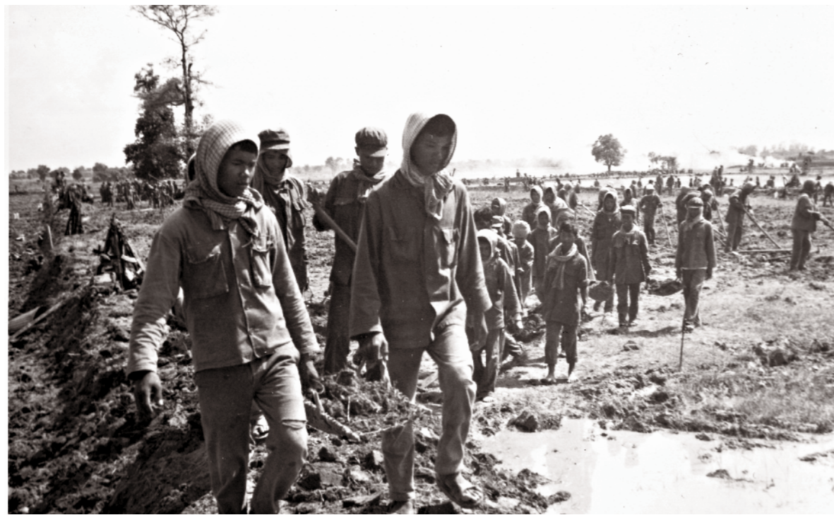
People working at a worksite during the Khmer Rouge regime (circa. 1975-1978). (Documentation Center of Cambodia Archives)
